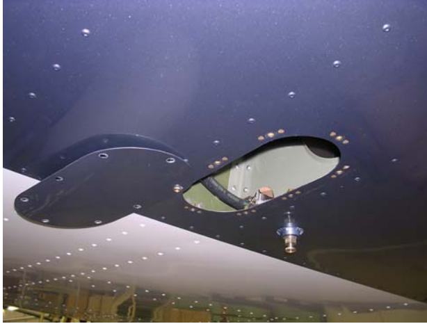
Picture 3 – inspection cover
